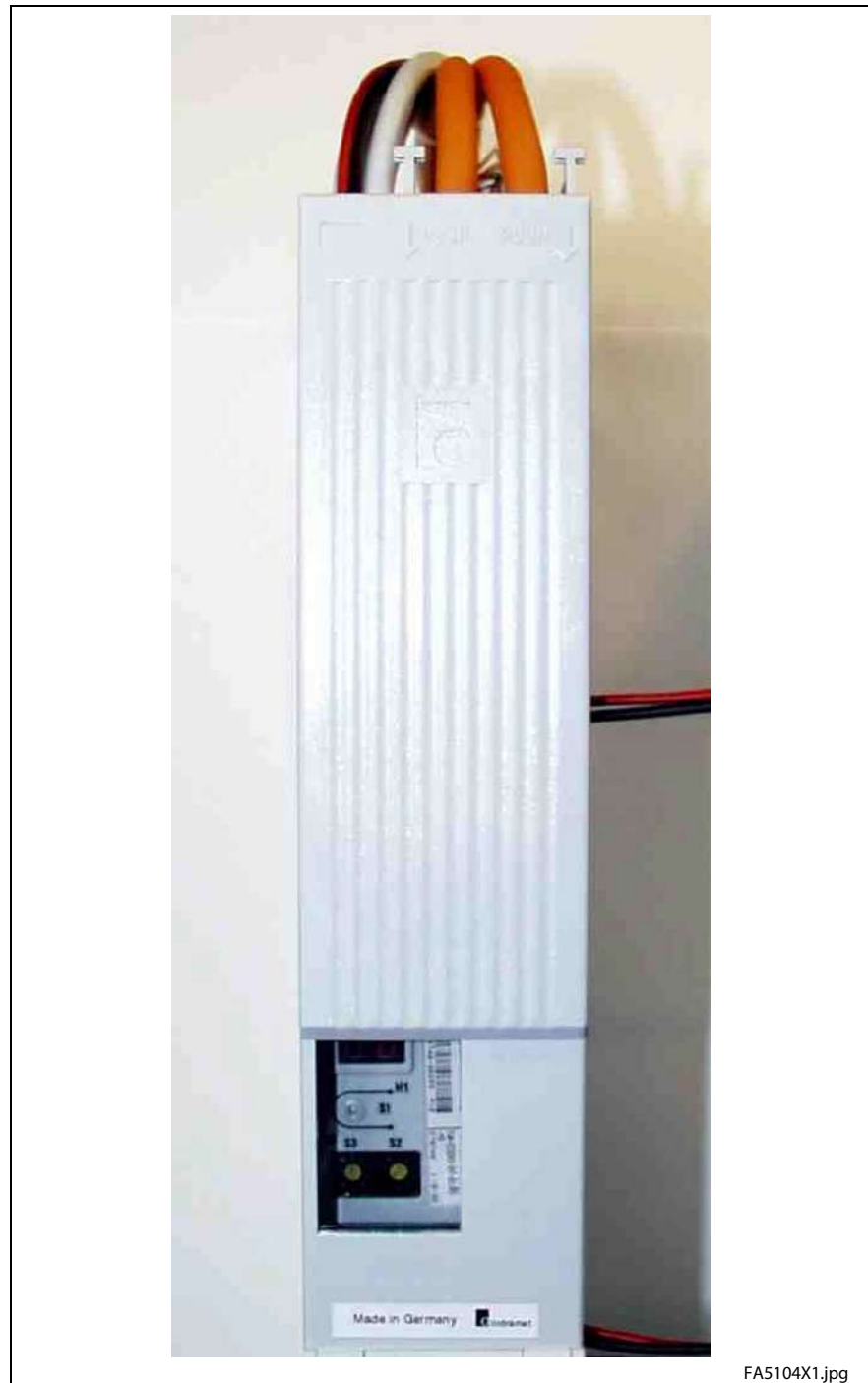
Fig. 16-21: View with contact protection
